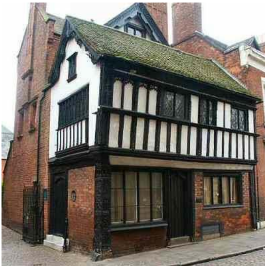
Ornate: the timber-framed Bayley House at No.22 and the brick-faced No.23 next door
